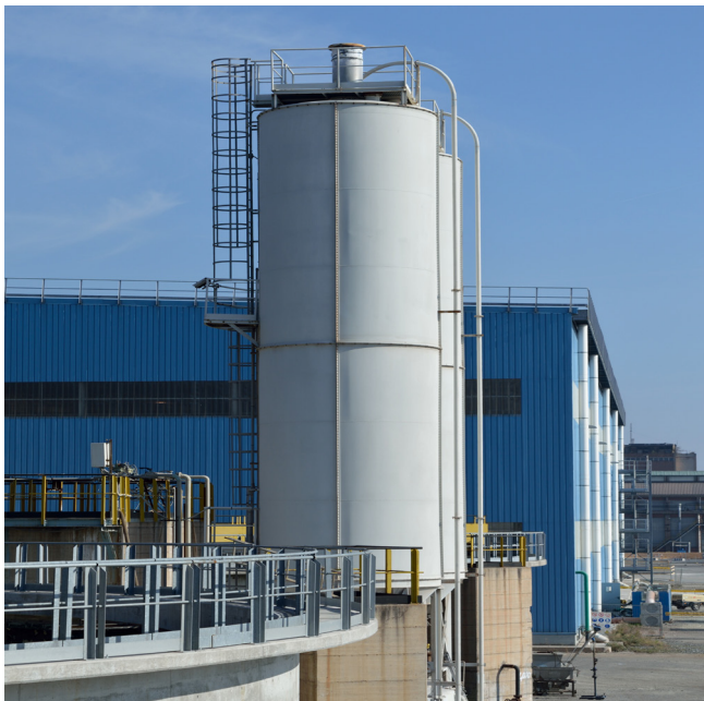
Figure 1. An example of one of the flour silos that needed to be replaced at this baking facility.
